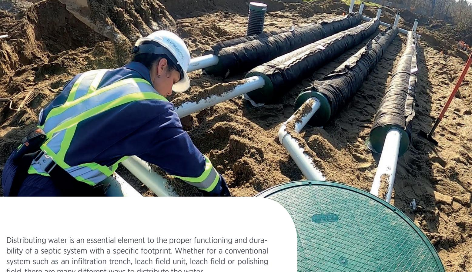
Distributing water is an essential element to the proper functioning and durability of a septic system with a specific footprint. Whether for a conventional system such as an infiltration trench, leach field unit, leach field or polishing field, there are many different ways to distribute the water.
