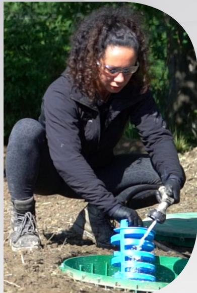
First, a clogged effluent filter will stop water from leaving the septic tank from its intended exit. This will make the water level rise inside the tank. If this situation continues, the water level could rise sufficiently for the fat, oil and grease that float on top of the water level and some suspended solids to flow over the effluent filter to reach the treatment unit.
